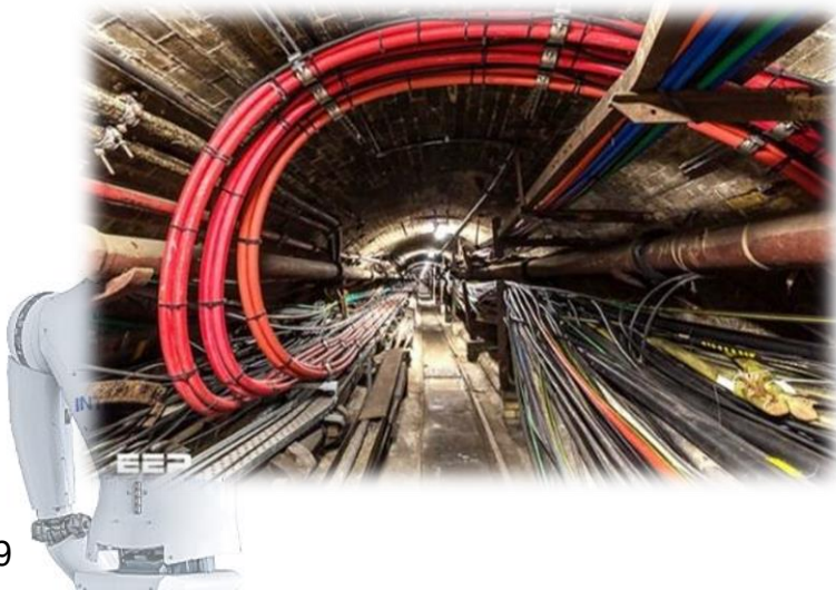
Underground Cable Project
